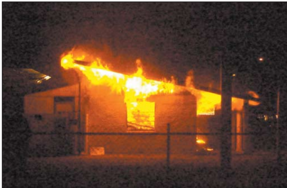
The Monday, May 3, fire at 2152 W. Apache Trail was an accident, said Apache Junction Fire District Fire Marshal Dave Montgomery. Photo by Raquel Ramirez.
